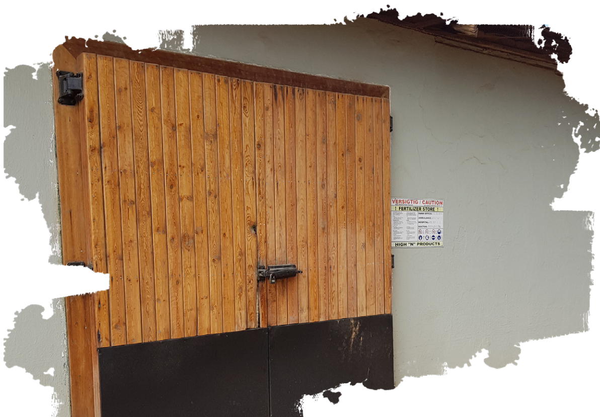
Entrance to chemical storage area
