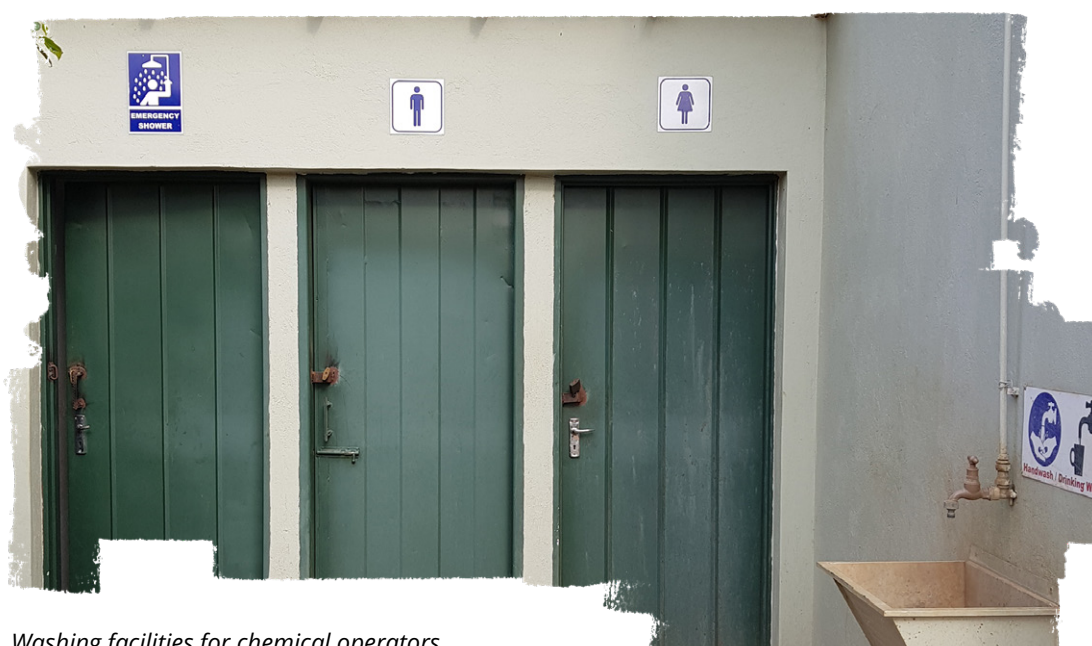
Washing facilities for chemical operators
